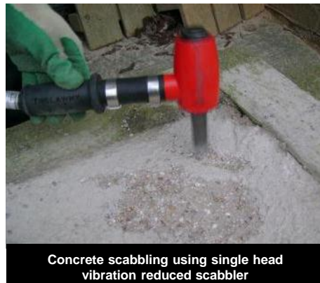
Concrete scabbling using bush hammer piston
